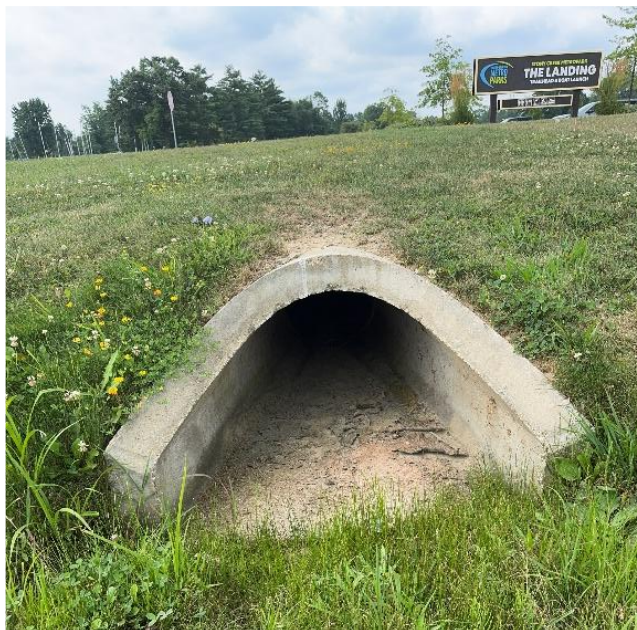
Figure 1: One of the many infrastructure points that are surveyed annually as part of our MS4 permit.
