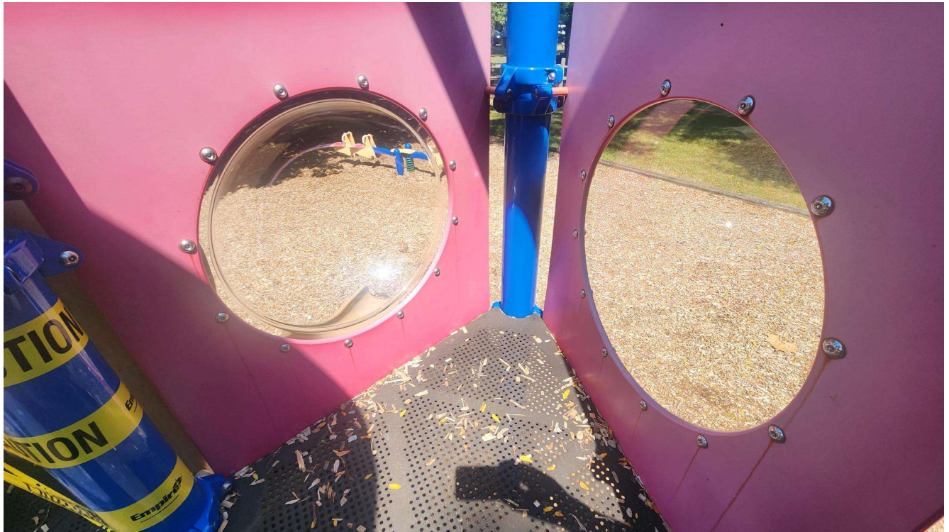
After: Window replacements at Delhi Playground, taken August 2026
