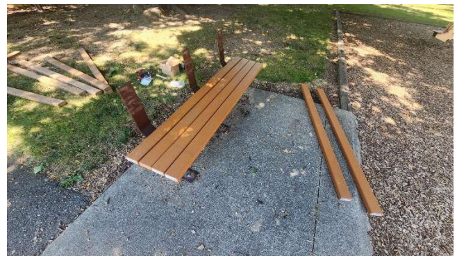
After: New bench slats arrived to be installed
