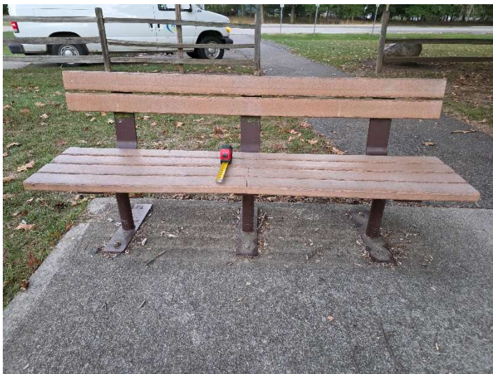
Before: Delhi bench is cracked
