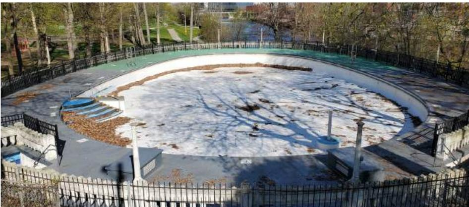
Moores Park Pool originally opened in August of 1922. Designed by former Lansing Engineer Wesley Bintz, the pool is seen as an irreplaceable asset in the local community. It's the oldest surviving pool of the 150 he designed across the country. Constant leaks and other unsafe conditions caused the pool to close indefinitely in 2019.
