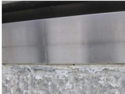
Image 19: 3/8" Gutter Return Tube Inlets
