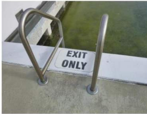
Image 22: Deep End Ladder Rails
