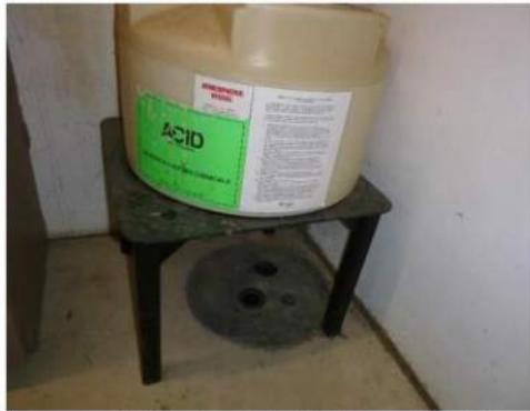
Image 69: Muriatic Acid Storage Tank & Stand
