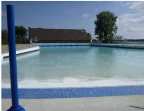
Image 86: Water Shy of Beach Entry Gutter
