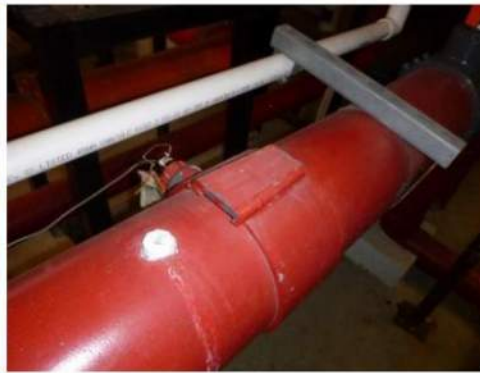
Image 48: Flow Meter Sensor
