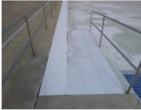
Image 20: Ramp Entry and Barrier Railing
