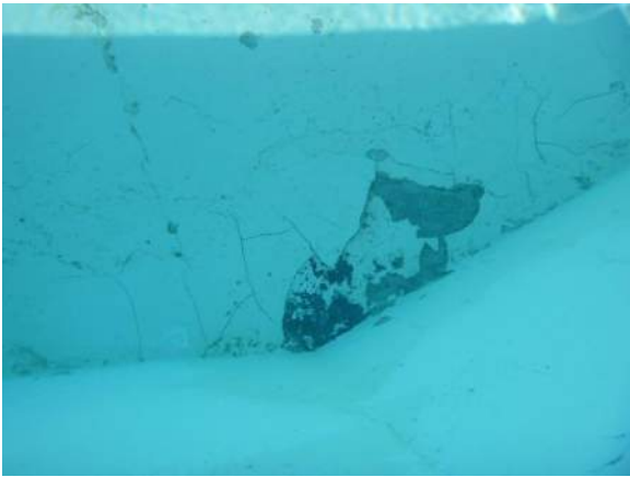
Pool cracking
