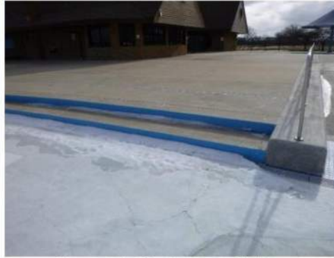
Image 25: Beach Entry Stairs
