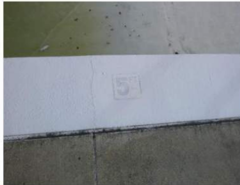
Image 27: Faded Depth Marking
