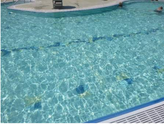
Expansion joint in pool area
