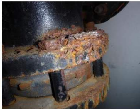
Image 38: Valve Corrosion
