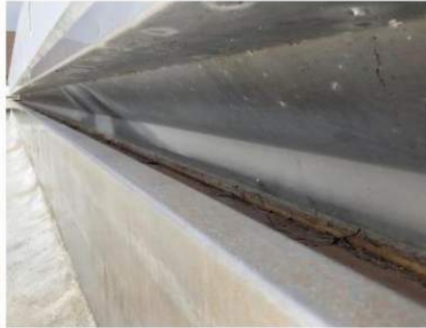
Image 14: Interior Gutter Channel Profile
