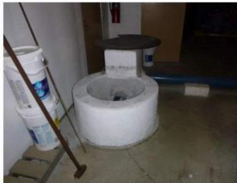
Image 52: Sanitary Waste Pit
