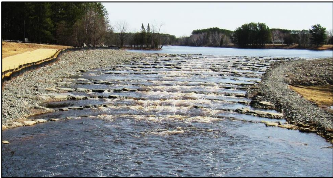
Figure 14 : Looking Upstream at a Completed Rock-Arch Rapids Project Designed by Dr. Aadland on the Willow River of Minnesota
