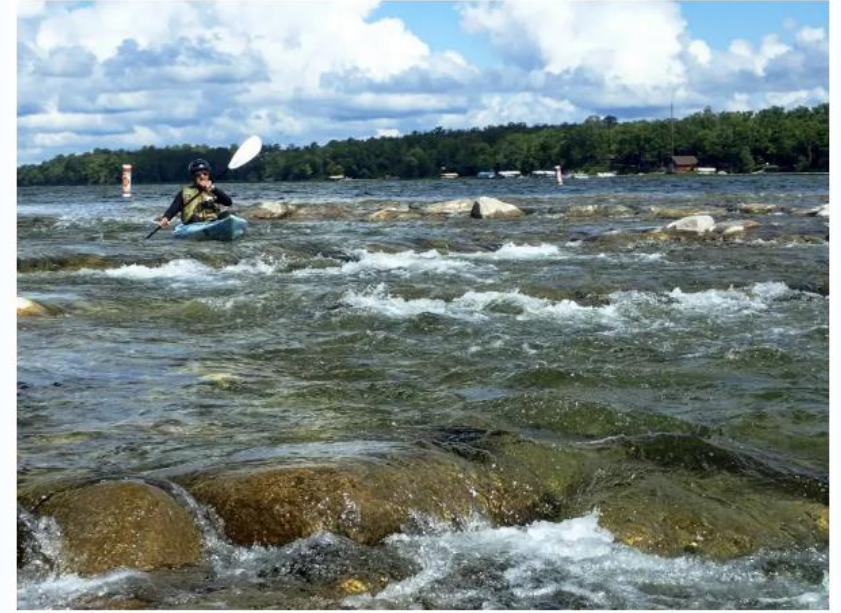
A kayaker paddles down Knutson Dam rapids on Cass Lake in Minnesota. The 2015 project removed the failing Knutson Dam and reconnected the Mississippi River at the outlet of Cass Lake with rock arch rapids, restoring spawning habitat for warm-water species such as walleye and white sucker. Courtesy of Minnesota DNR
