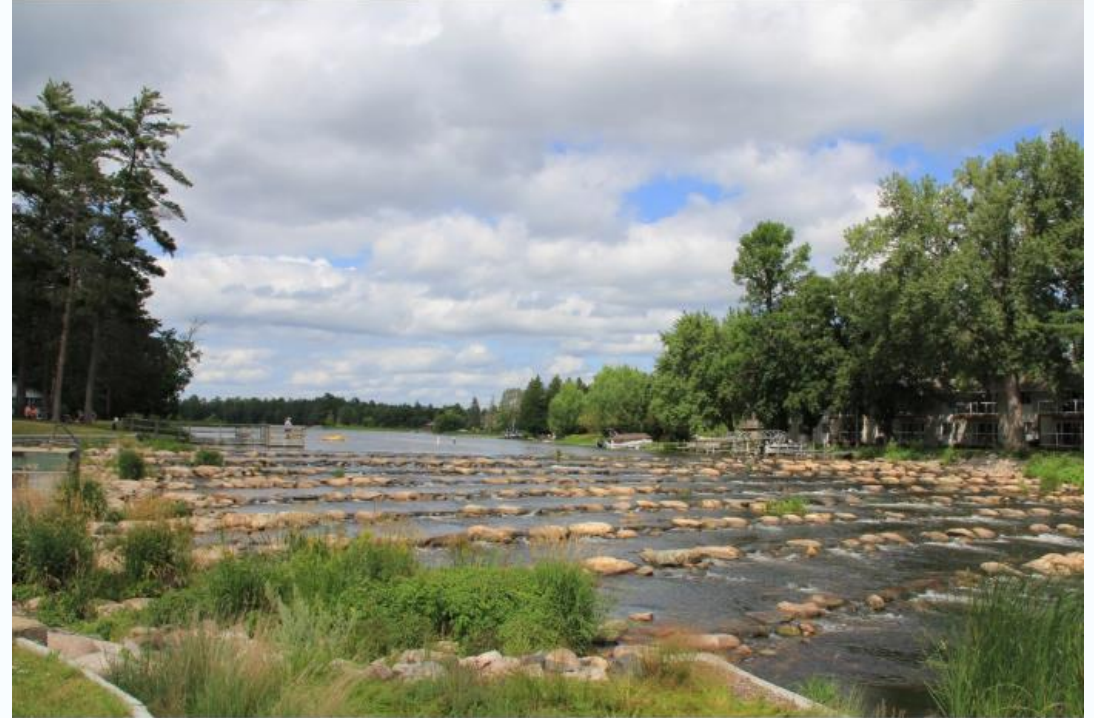
This rock riffle in Pine River replaced a traditional dam built in 1910 to hold back water flowing from Norway Lake into the Pine River. The old dam was designated as "high hazard," thus in need of replacement. (Minnesota Prairie Roots copyrighted photo July 2024)
