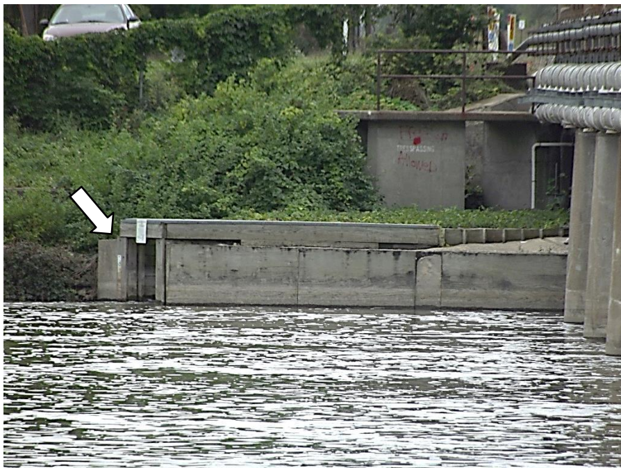
Photograph 8 – Downstream right principal spillway abutment wall. Note the outlet of the fish ladder.
