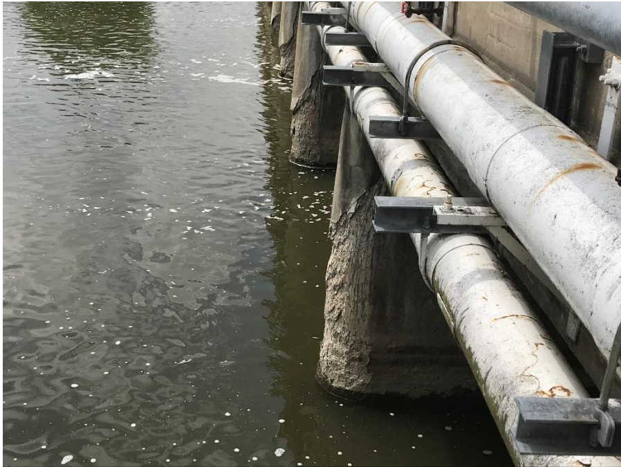
Photograph 15 – Typical pier spalling and delamination
