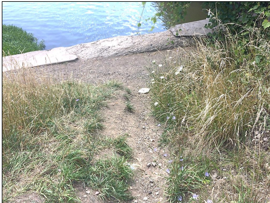
Photograph 6 – Downstream face of left abutment viewed from left Note the foot traffic erosion
