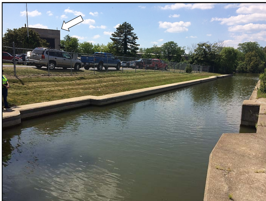
Photograph 6 – Earthen needle section located between lock and powerhouse Note the arrow indicating the location of the former powerhouse
