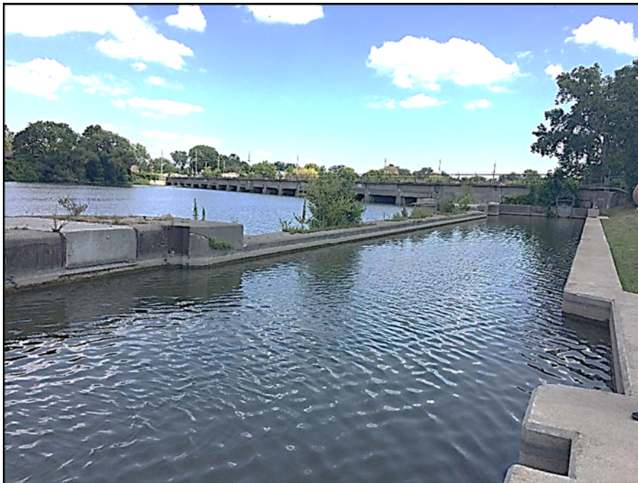
Photograph 15 – Abandoned lock viewed from upstream Note that the right wall was recently reconstructed
