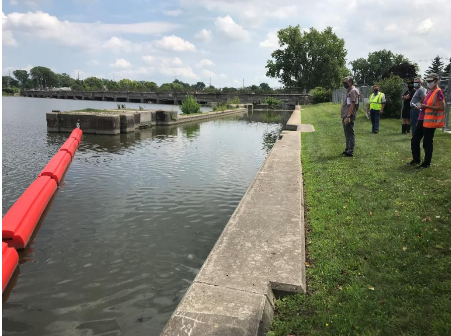
Photograph 16 – Right abutment wall of abandoned lock
