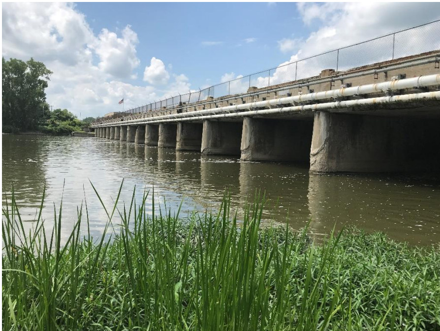
Photograph 14 – Downstream face of bridge over spillway Note the spalling and delamination of piers
