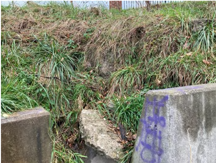
Photo #34: Embankment Downstream Slope. Right above storm sewer from Rhodes. likely from seepage observed. Issue: Depression, Action: Maintenance.
