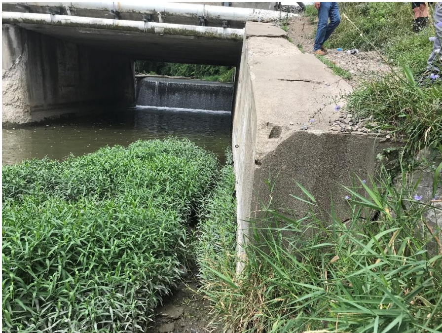
Photograph 12 – Left downstream abutment wall Note the spalling
