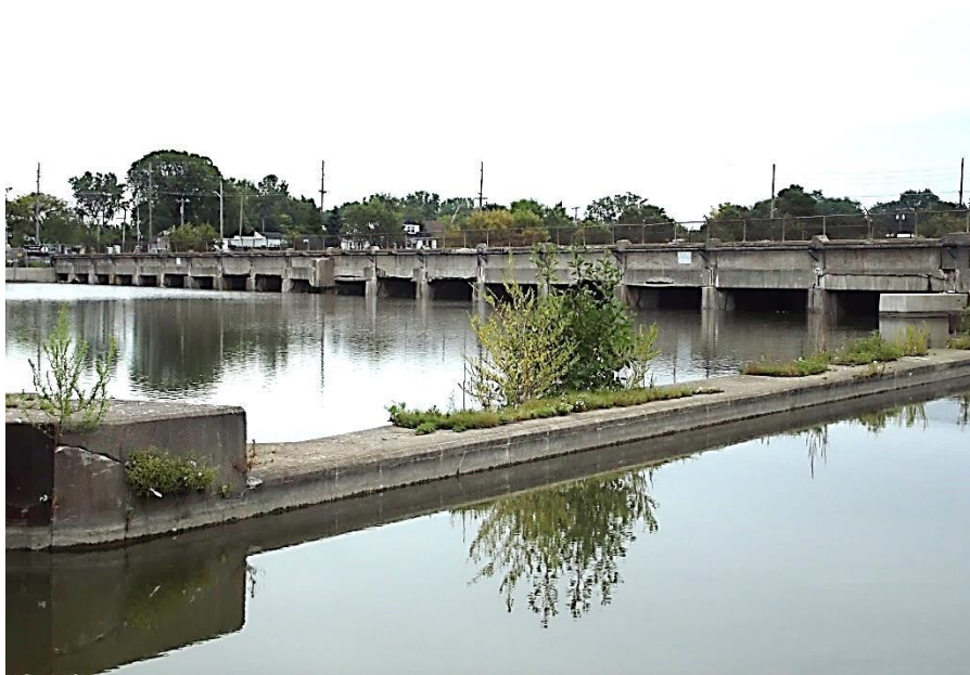
Photograph 13 – Downstream portion of lock wall viewed from right. Note the deteriorated concrete and vegetation growing from cracks.
