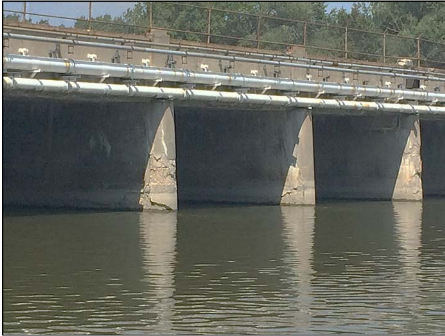
Photograph 13 – Typical spalling of bridge piers
