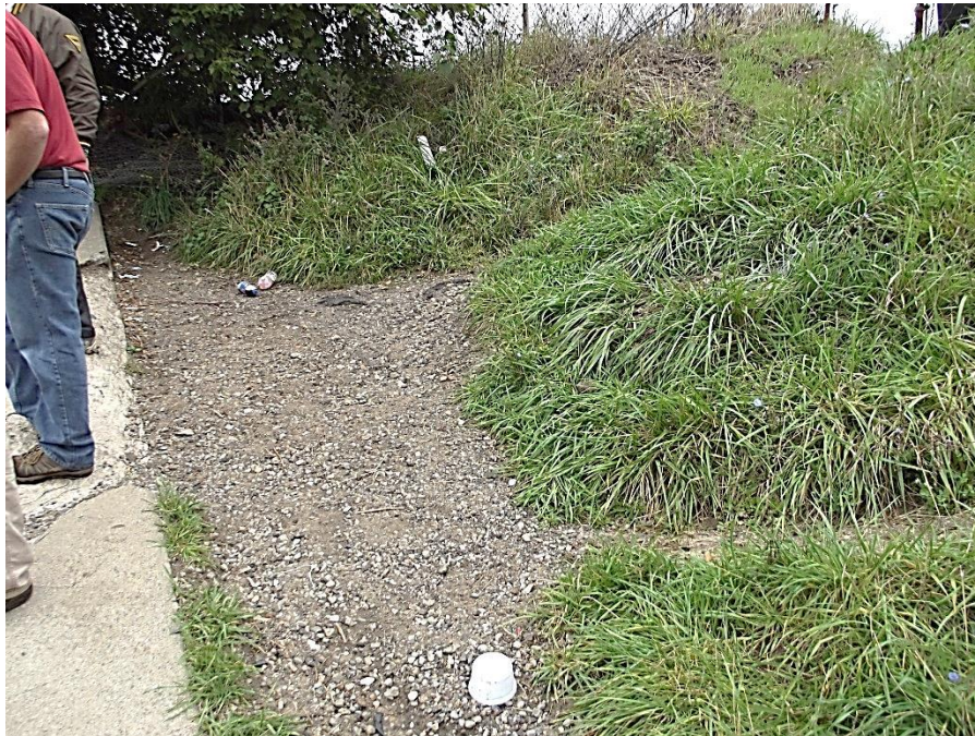
Photograph 5 – Downstream face of left embankment viewed from left. Note the foot traffic erosion.
