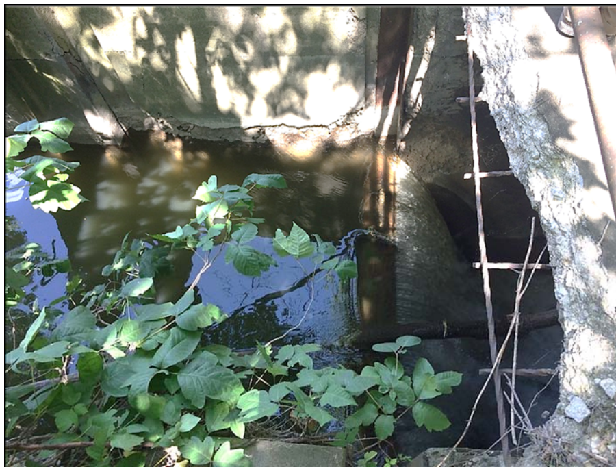
Photograph 20 – Small powerhouse head gate viewed from right Note the deteriorated concrete and exposed reinforcing steel
