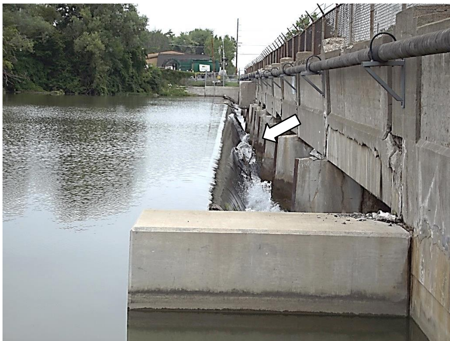
Photograph 6 – Principal spillway crest viewed from right. Note the minor debris build up.
