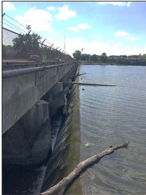
Photograph 7 – Principal spillway crest viewed from left Note the minor buildup of woody debris
