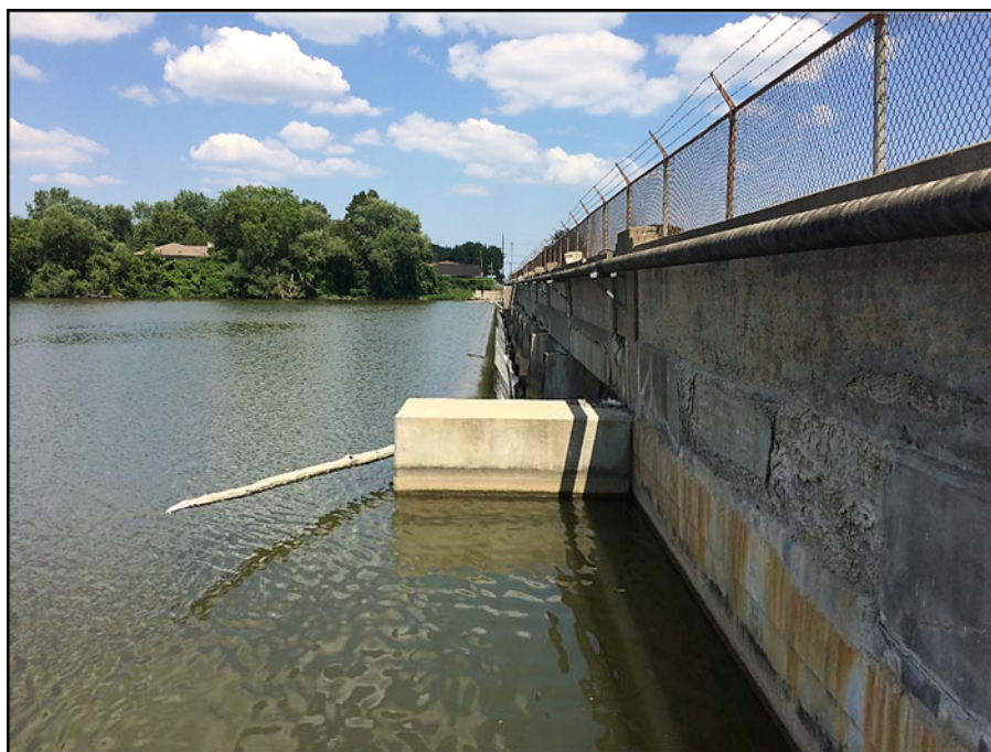
Photograph 10 – Upstream right spillway abutment wall Note that a portion of this wall was recently reconstructed
