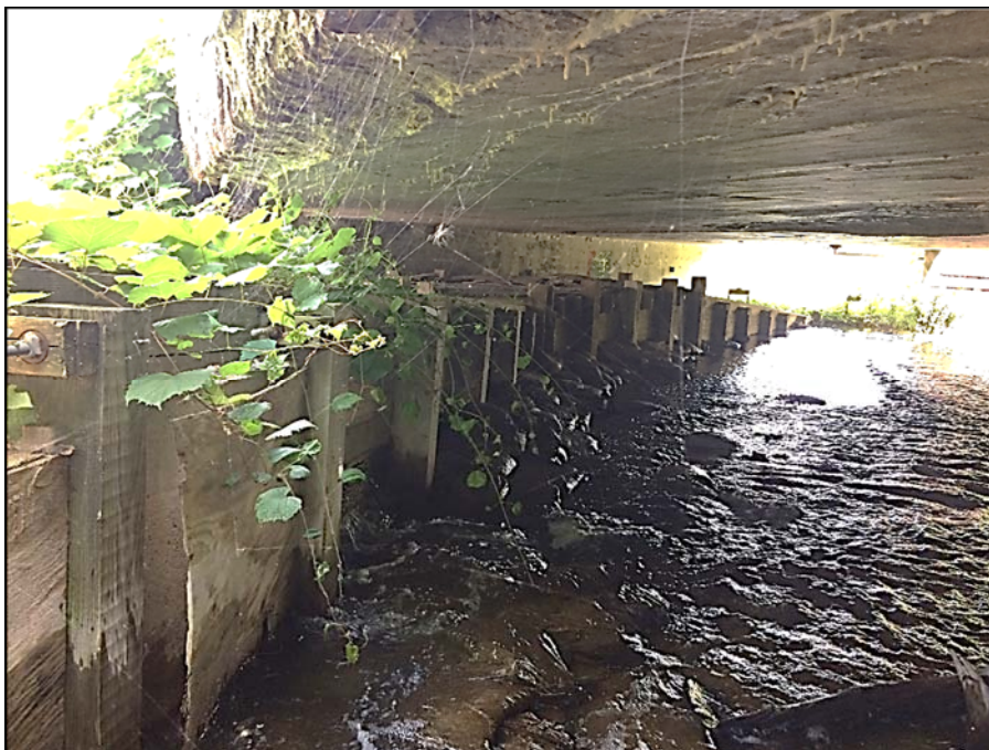
Photograph 18 – Wooden fish ladder viewed from upstream
