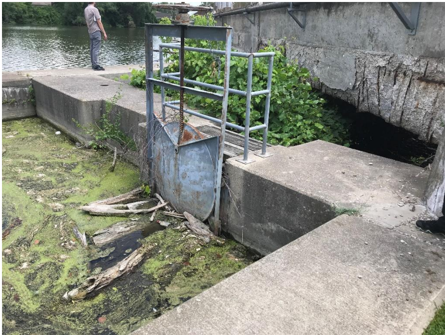
Photograph 18 – Right lock gate and operator Note that this gate acts as the inlet to the DNR fish ladder
