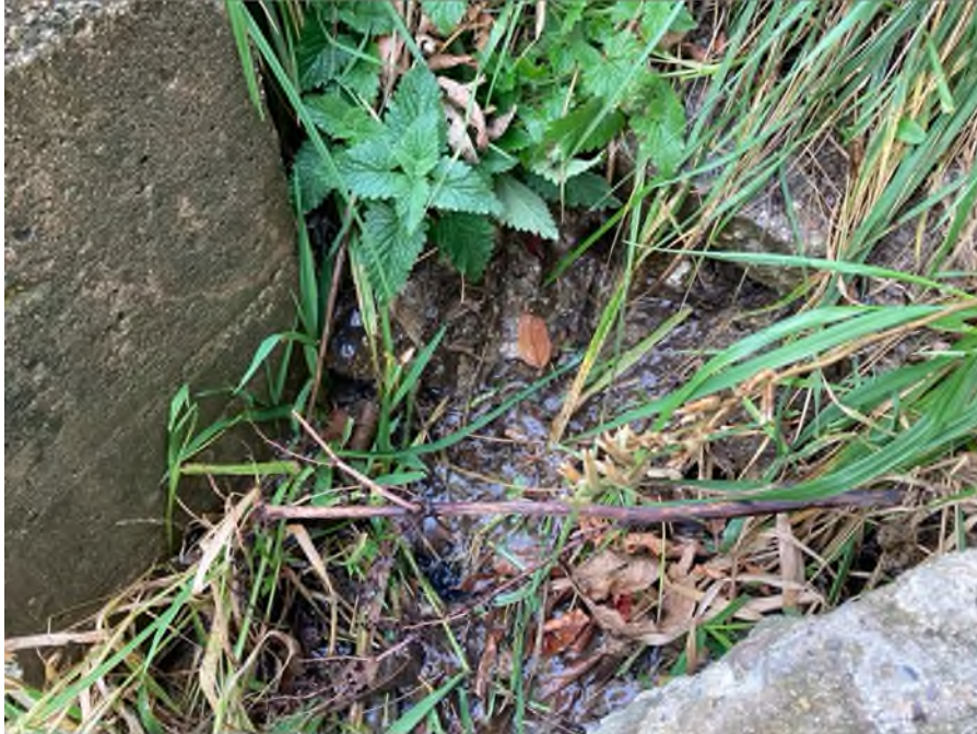
Photo #33: Embankment Downstream Slope. Might be from storm sewer. Issue: Seepage, Action: Monitor. Type: Flow.
