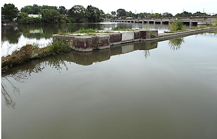
Photograph 12 – Upstream portion of lock wall viewed from right. Note the deteriorated concrete vegetation growing from cracks.
