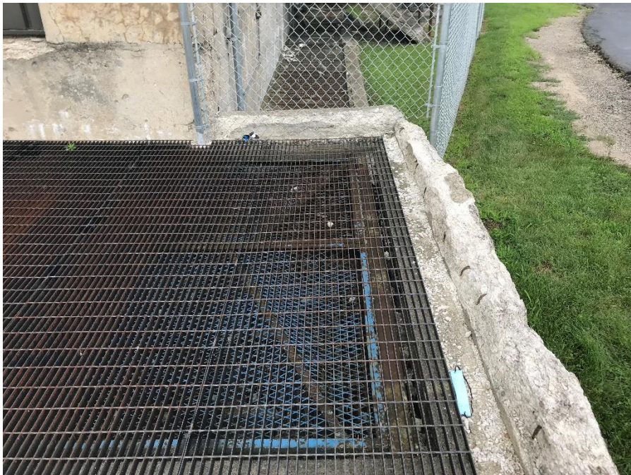
Photograph 24 – Bypass channel at left of powerhouse Note that there was flow through this channel during this inspection
