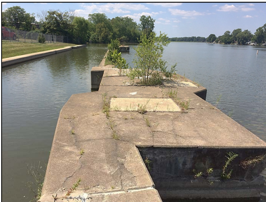
Photograph 17 – Left wall of abandoned lock Note that this is the original wall and shows signs of deterioration
