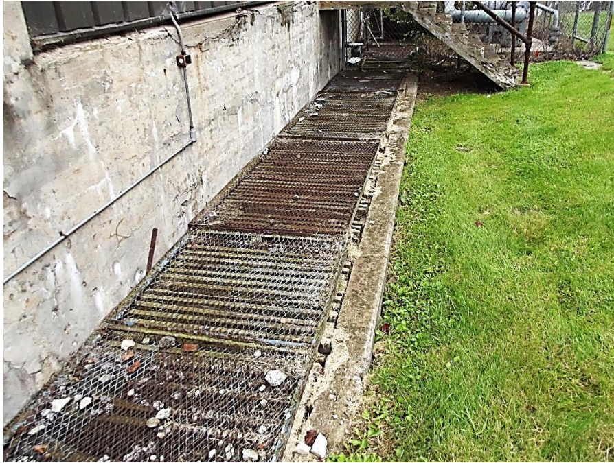
Photograph 19 – Channel along right powerhouse wall. Note that there was flow through this channel on the date of the inspection.
