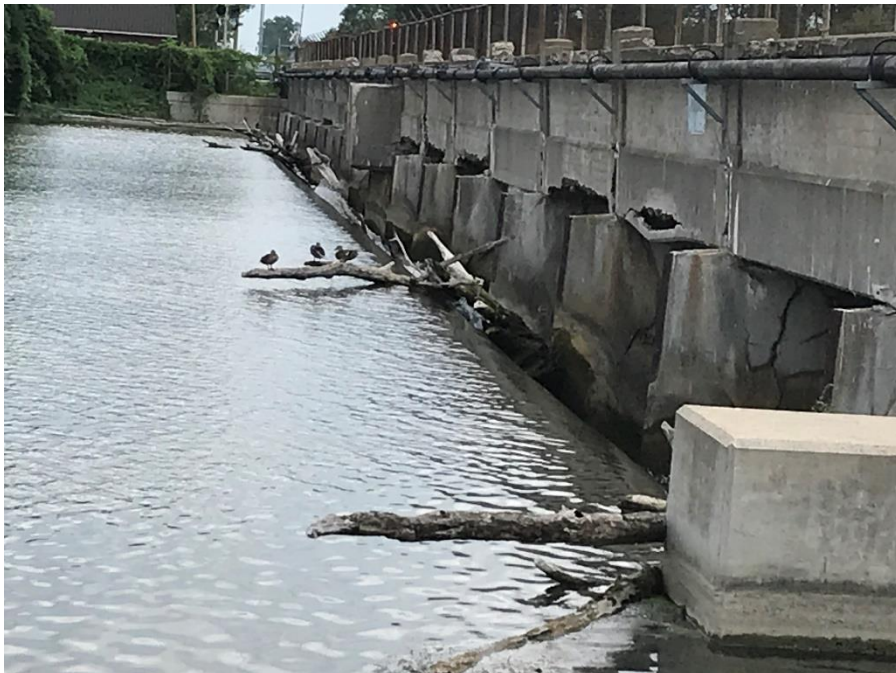
Photograph 8 – Spillway crest viewed from right Note the minor debris build up and delamination of bridge beams
