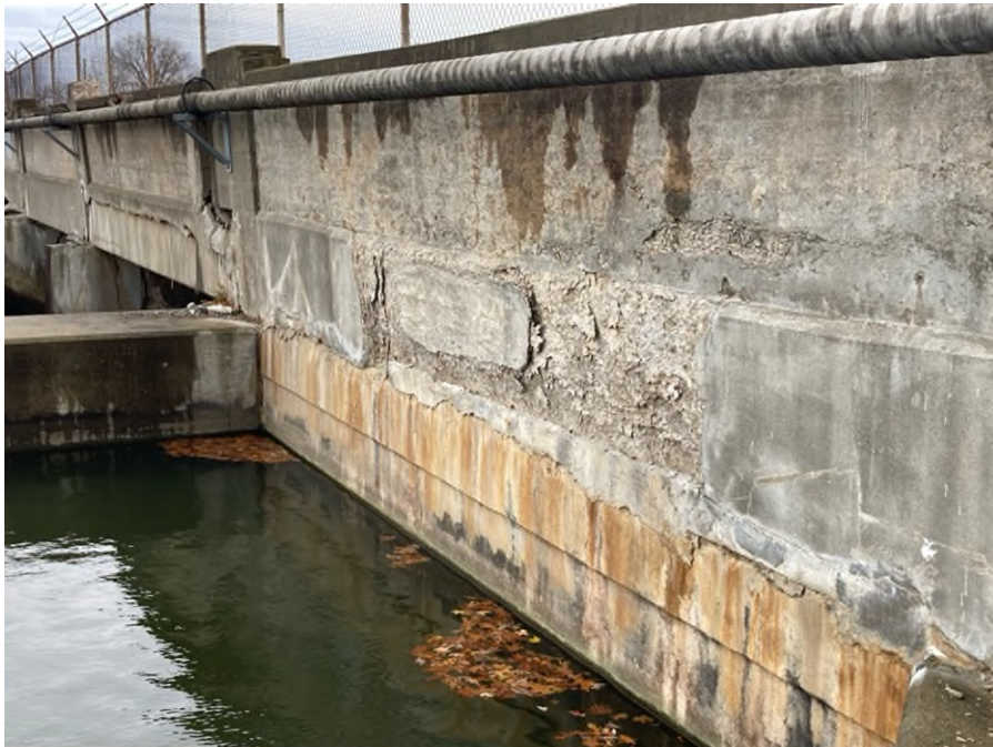
Photo #9: Principal Spillway Abutment Right Wall. Issue: Deteriorating Material, Action: Maintenance. Material: Concrete.
