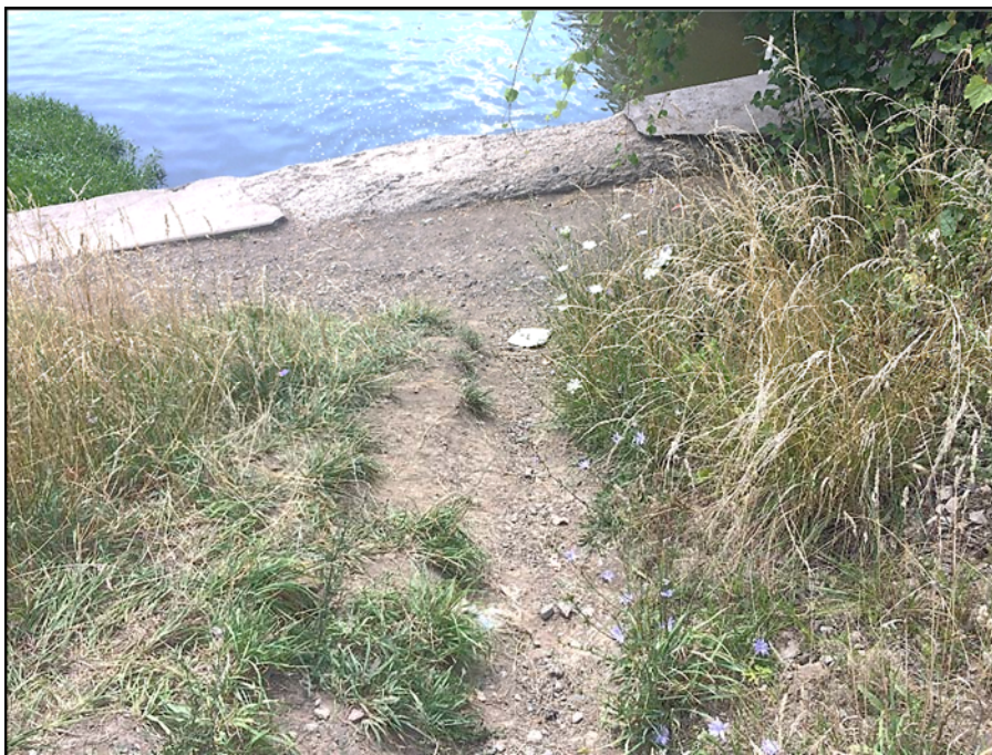
Photograph 4 – Left abutment viewed from left Note the foot traffic erosion
