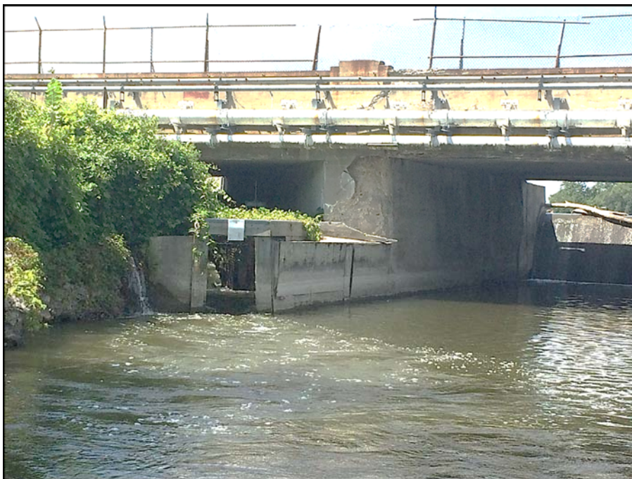
Photograph 11 – Downstream right spillway abutment wall Note the spalling and fish ladder outlet
