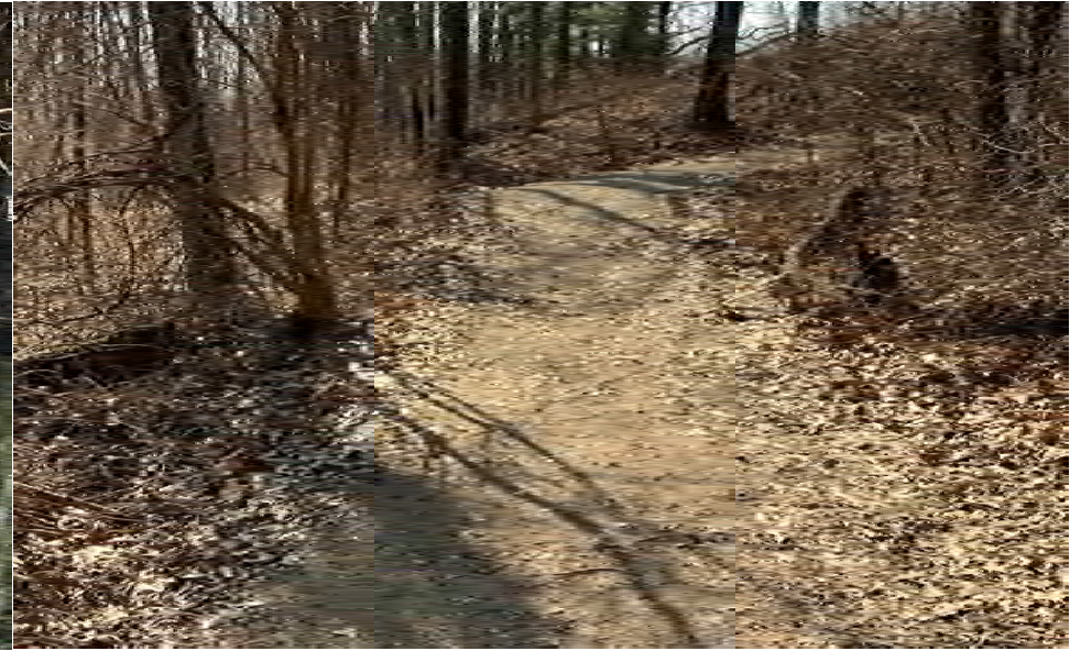
#18. (Facing Southeast): Adjust grade of existing aggregate paths. The 6' & 8' wide UA 21AA aggregate paths with limestone fines shall not exceed 5% running slope & 2% cross pitch.
