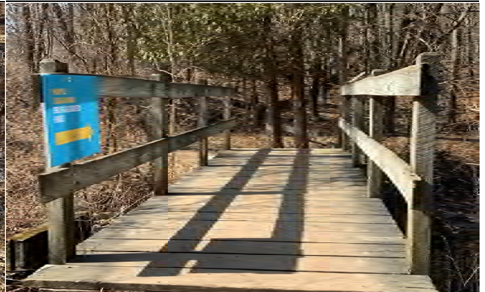
#14. (Facing South): Adjust grade of existing path. Realign the existing trail. The UA path shall be min. 6' wide & constructed of 21AA aggregate with limestone fines.
