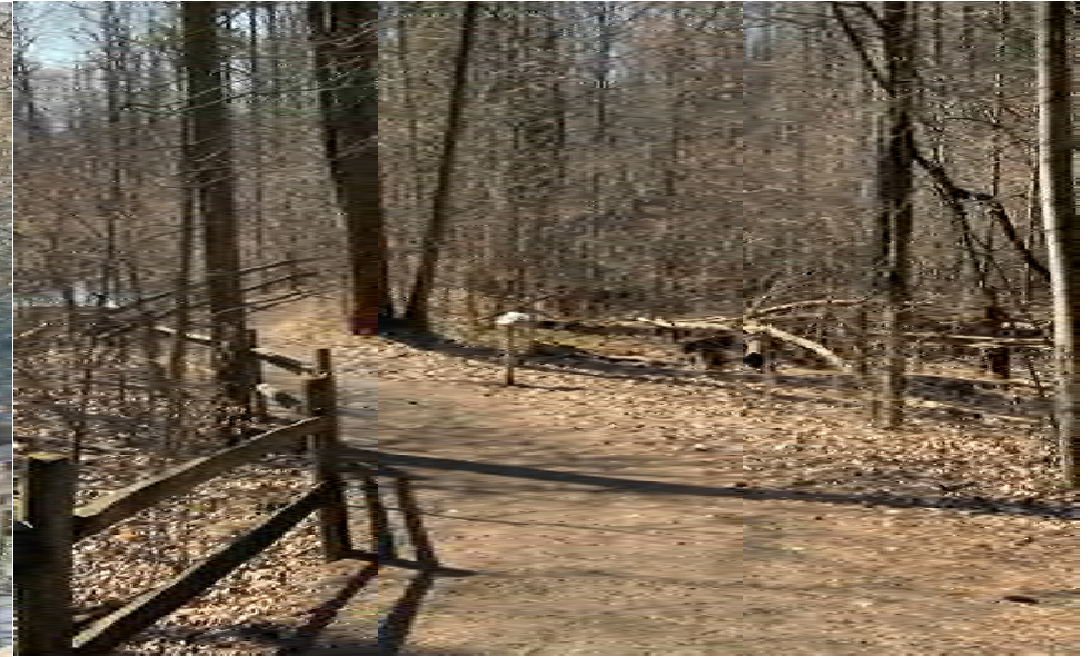
#14. (Facing South): Adjust grade of existing path. Realign the existing trail. The UA path shall be min. 6' wide & constructed of 21AA aggregate with limestone fines.
