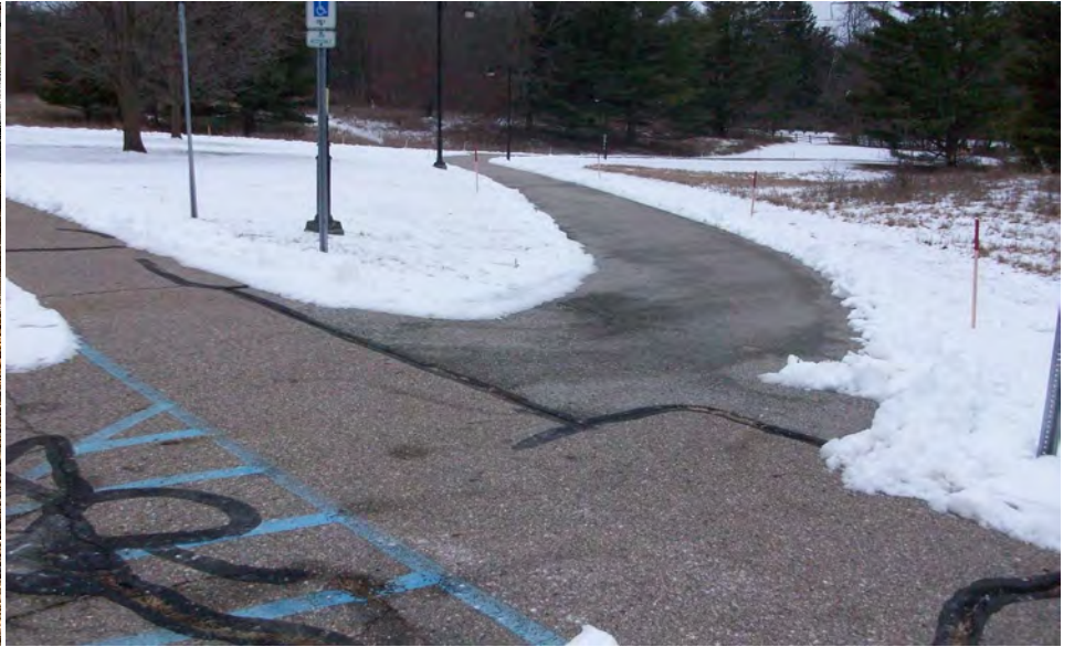
#22. (Facing Southwest): The steep section of walk down to the Nature Center will be reconstructed to meet UA design standards. The running slope ( \pm 6\% ) and cross slopes ( \pm 4\% ) exceed ADA standards at this time.
