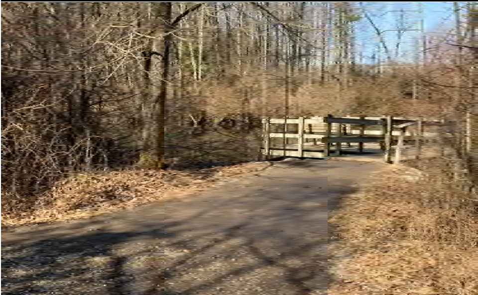
#11. (Facing West): Adjust width & grade of existing path to new overlook. The short UA paths shall be 6' wide & constructed of 21AA aggregate with limestone fines. Transition onto the platform shall not exceed 1/2".
