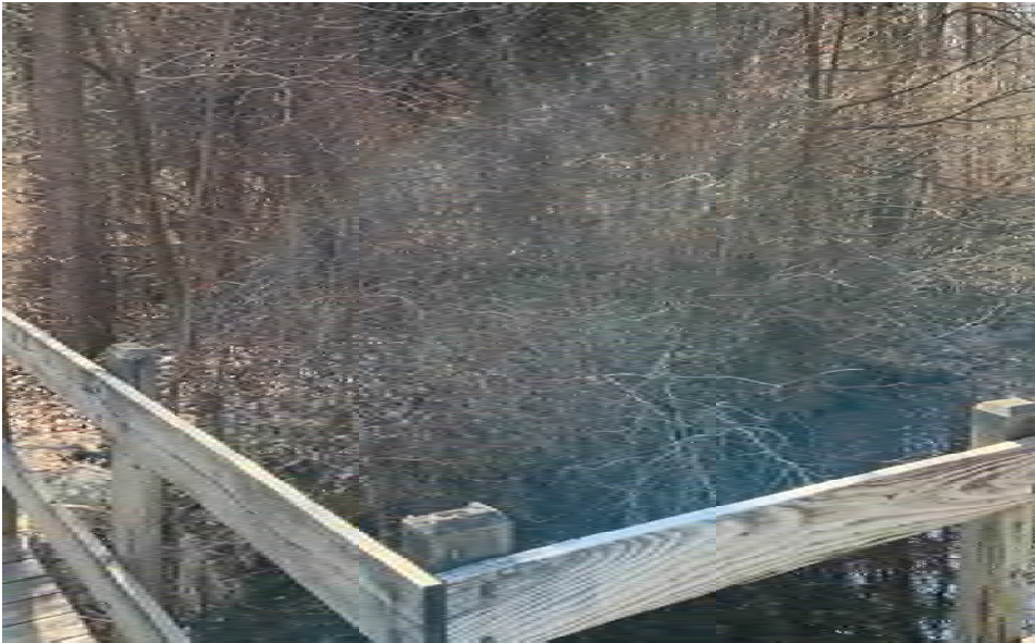
#13. (Facing East): 10' X 30' overlook structure with wheelchair guards to be added along bank. Proposed transitions on to the platform shall not exceed 1/2".
