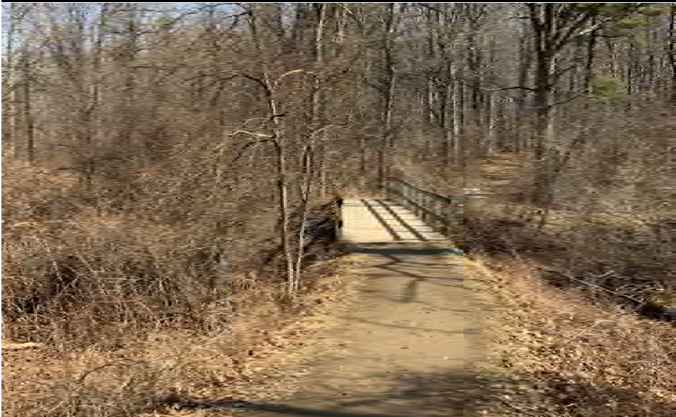
#19. (Facing Northeast): Replace bridge #3 with a prefabricated bridge with railings. Transitions onto bridge shall not exceed 1/2".
