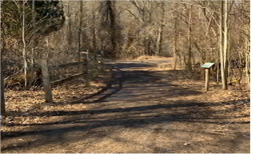
#10. (Facing Southwest): Adjust grade of existing aggregate path. The 6' & 8' wide UA 21AA aggregate paths with limestone fines shall not exceed 5% running slope & 2% cross pitch.
