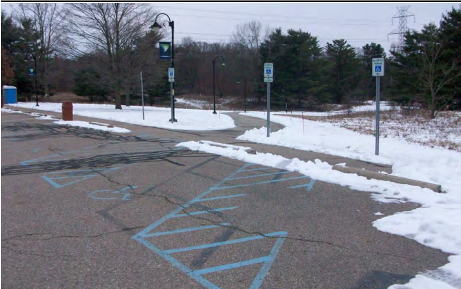
#23. (Facing Southwest): A portion of the asphalt lot will be reconstructed & restriped. Slopes within this section of lot shall not exceed 2% slope. A total of five van accessible spaces will be striped & signed. Each space will have its own striped aisle.
