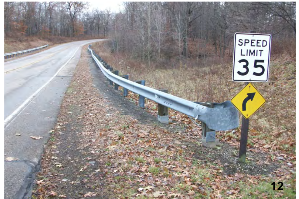
The west guardrail will be removed and reconstructed further east to create space for the trail. The roadway alignment needs to shift east requiring new pavement and resurfacing.
