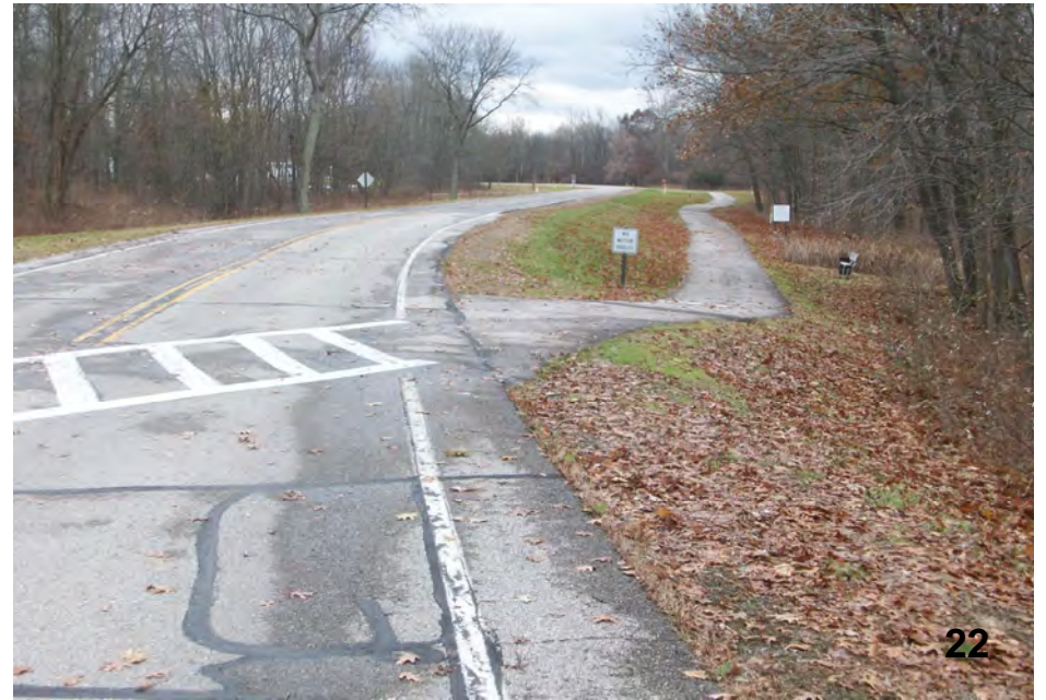
Portion of existing trail will be reconstructed. The segment near the crossing is too steep and does not meet ADA requirements.
