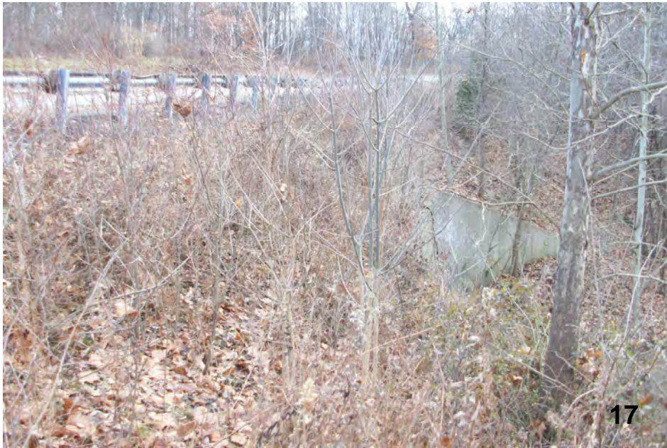
Guardrail to be replaced and shifted closer to the road creating room for the trail and wood safety fencing above the box culvert.
