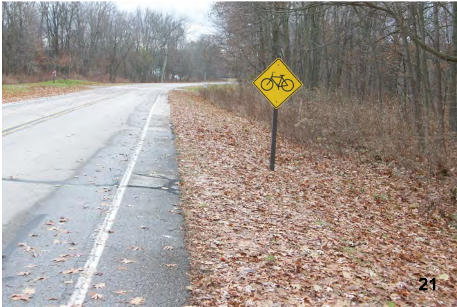
Existing crosswalk location to be moved. Crossing to be 90 degrees to road to improve safety. New signs to be installed.
