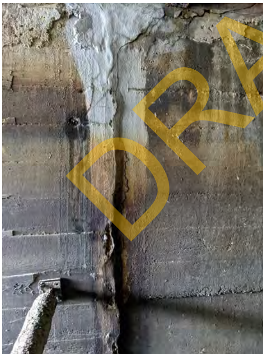
Photograph #8: Crack on North Wall
