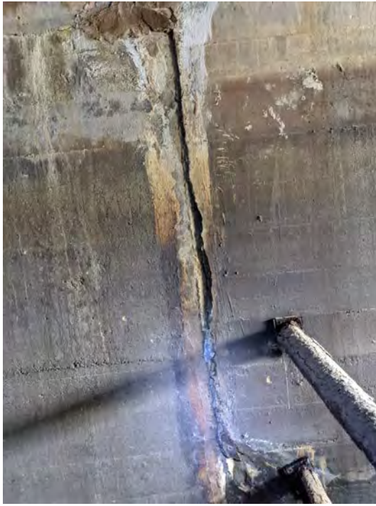
Photograph #7: Crack on South Wall of Headrace
