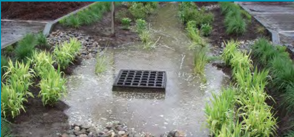
"Naturalized swale at Polk Valley Park." Stormwater BMPs, David Brandes, https://sites.lafayette.edu/brandesd/courses/ce-421/stormwater-bmps/ .
