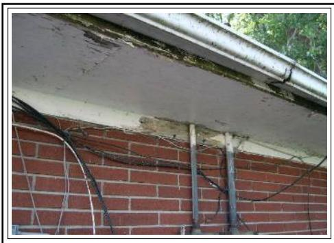
Peeling Paint & Unsecured Wiring
