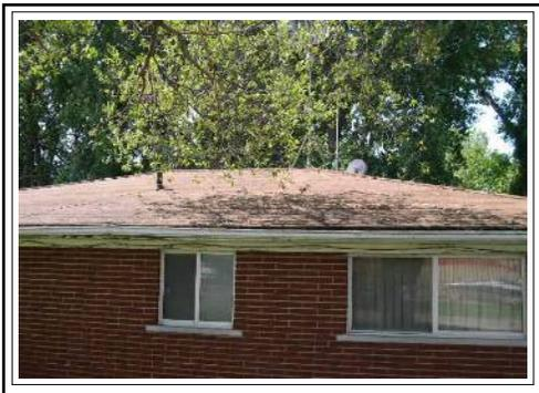
Peeling Paint, Unsecured Wiring, Roof Nearing the End of Useful Life
