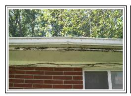
Damaged Gutters, Peeling Paint
