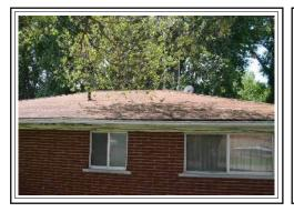
Peeling Paint, Unsecured Wiring, Roof Nearing the End of Useful Life
