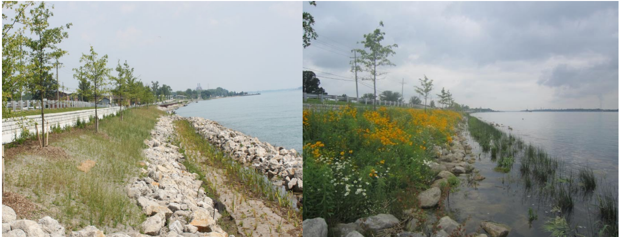
Restored Great Lakes Coastal Wetlands with detached breakwaters along the St. Clair River (project management, design and photos by GEI staff) at Marysville, Michigan on the St. Clair River
