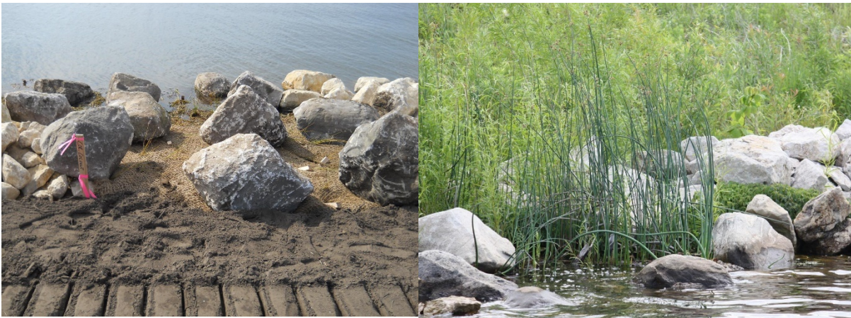
Restored High Energy Shoreline with Bioengineering and Rock Gaps (GEI, Muskegon Lake)
