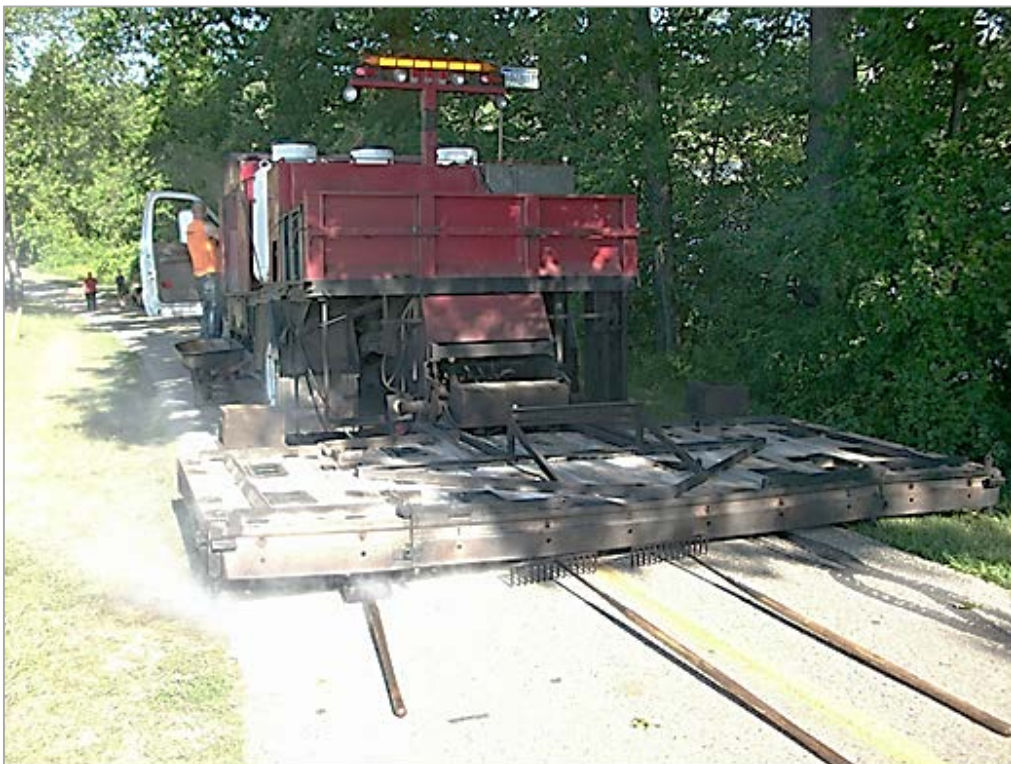
(2) Heating of asphalt
