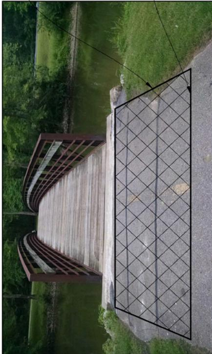
**REMOVE/REPLACE 10 LF OF ASPHALT PATH FROM EDGE OF ABUTMENT (PATH WIDTH VARIES APPROX. 10'-13') EACH SIDE OF BRIDGE**
