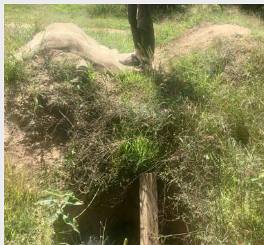
Open borrow pit hazard adjacent to a jump feature.
