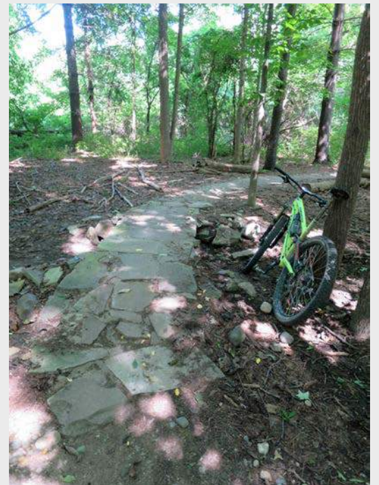
Rock armored tread that mitigates seasonally soft/muddy trail conditions.
