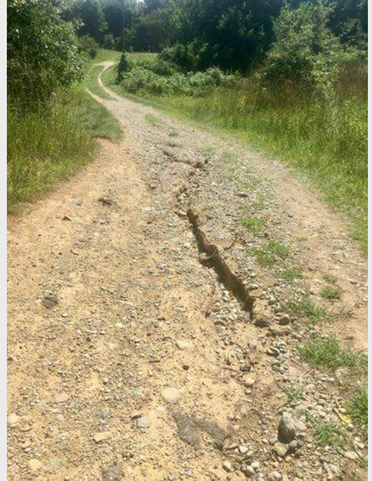
Rutting occurring on double track where drainage is not directed off the trail
