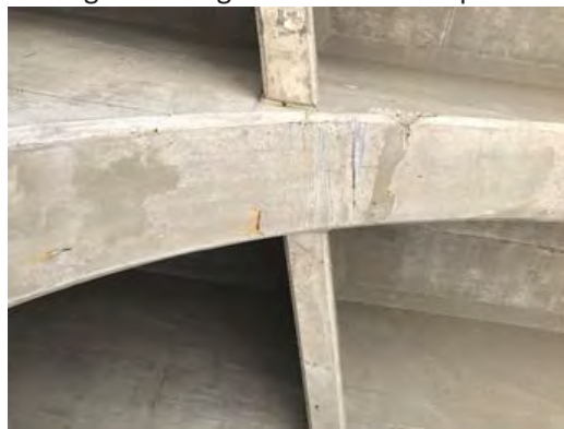
Damage from high load hits was repaired
