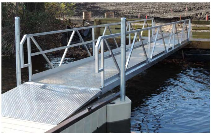
PROPOSED GANGWAY, HINGED AT TOP WITH TRANSITION PLATE AND ROLLERS AT BOTTOM FOR WATER FLUCTUATIONS.
