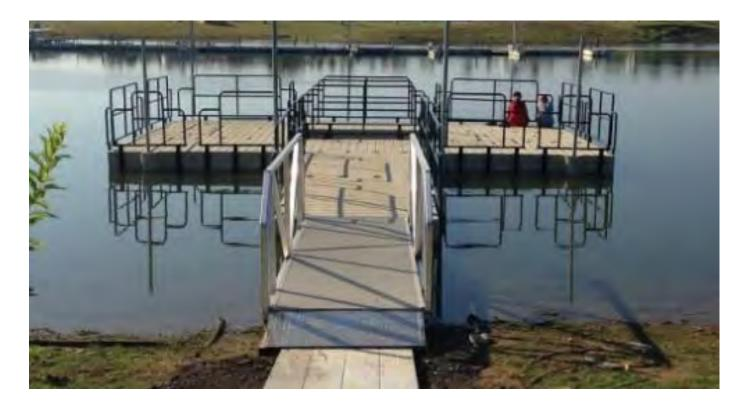
PHOTO SHOWING THE EZ DOCK STEPPED RAILING SYSTEM. A MINIMUM OF 25% OF THE RAILING ON THE FISHING PLATFORM WILL BE LOWERED FOR IMPROVED ACCESS TO THE WATER. SMALL GAPS BETWEEN RAILING SECTIONS WILL AID IN RETRIEVING A CAUGHT FISH.
