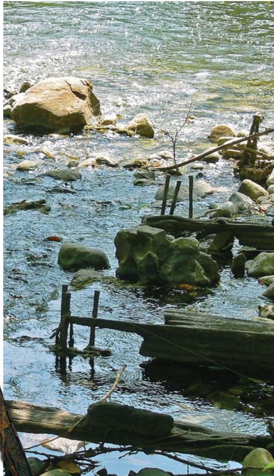
The remains of the Hudson Mill millrace.
